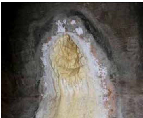
Picture 3 Drains choked with calcinations
